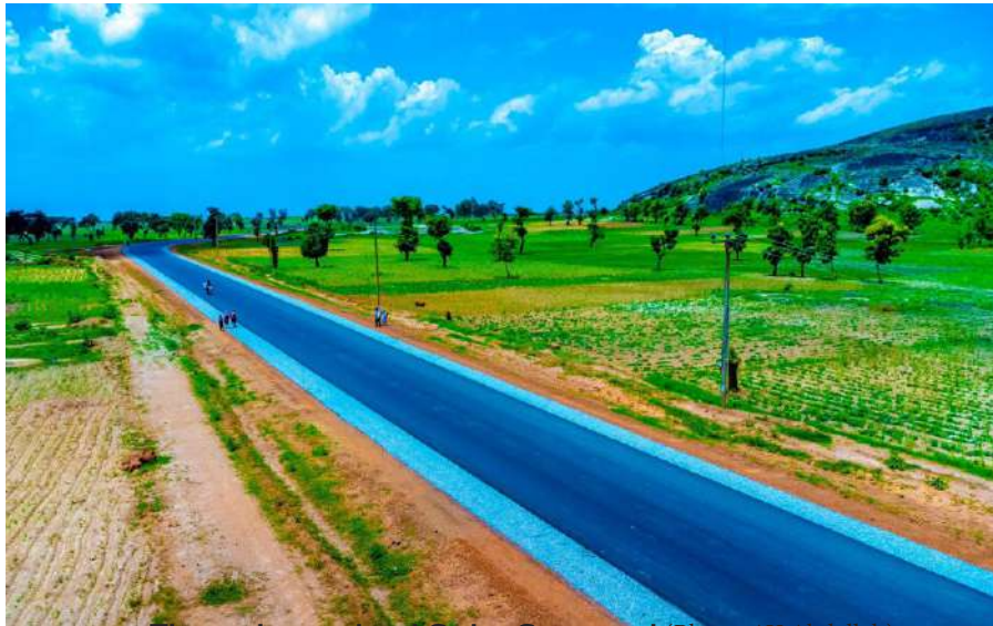
The newly completed Gadan Gayan road (Photo: AY Abdallah)
