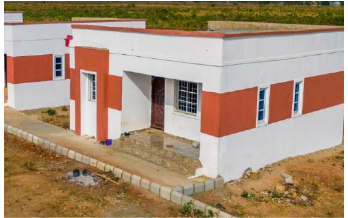
A typical house in the estate given free to the displaced persons
