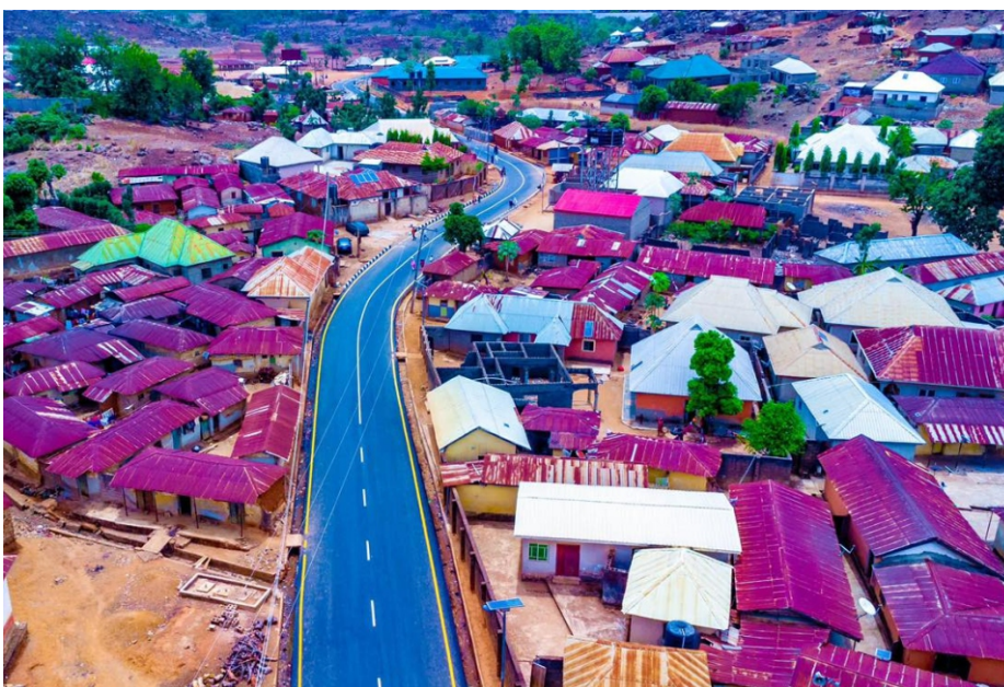
Some of the completed roads in Kagarko
