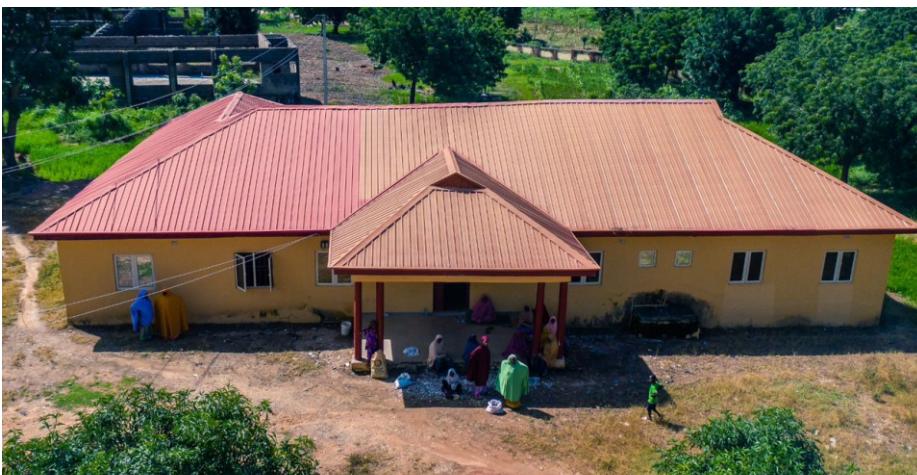
Some facilities at the Panpegua campus (above and below)awaiting commissioning
